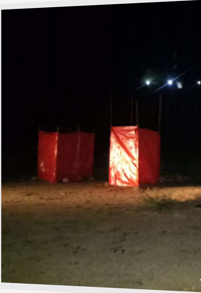
Installed 03 pit latrines at IRC High School Kotdiji
